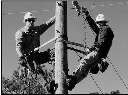
Electric Power Station Repairman Average salary = $65,230/year
